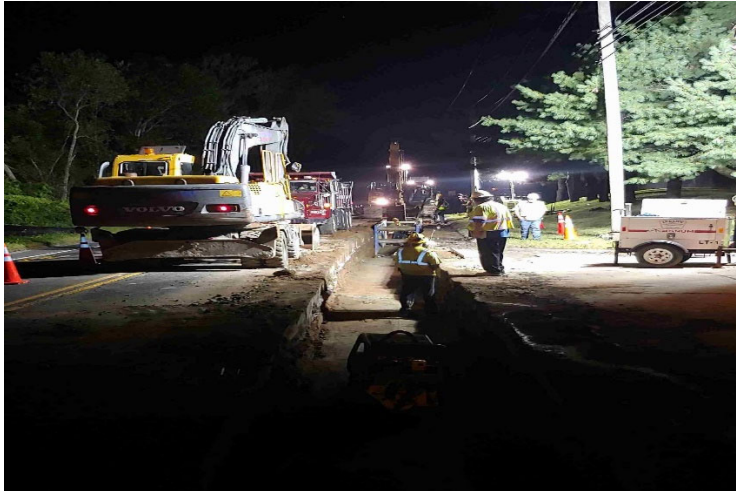
Installing 16" DIP pipe on RT. 17, Middletown
