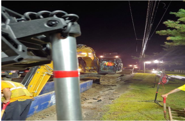
Installing 16" DI pipe on Rt 17, Middletown
